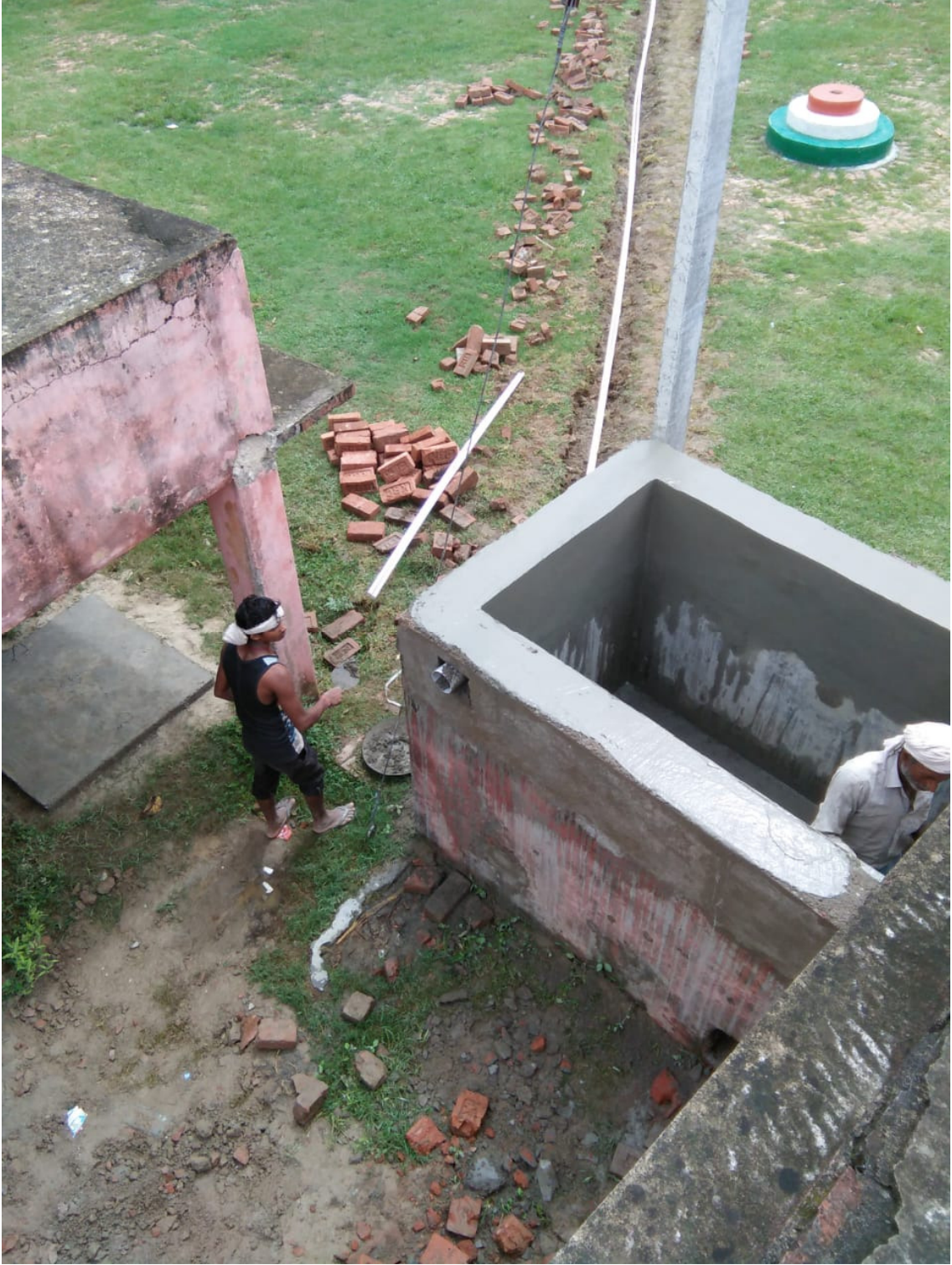
Finishing of tank
