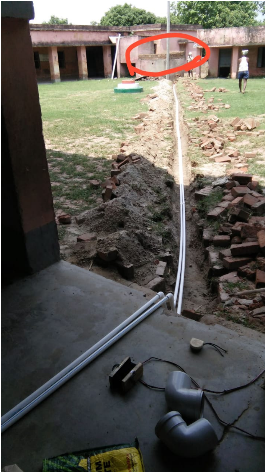
Increase the tank capacity and the pipe has also been laid
