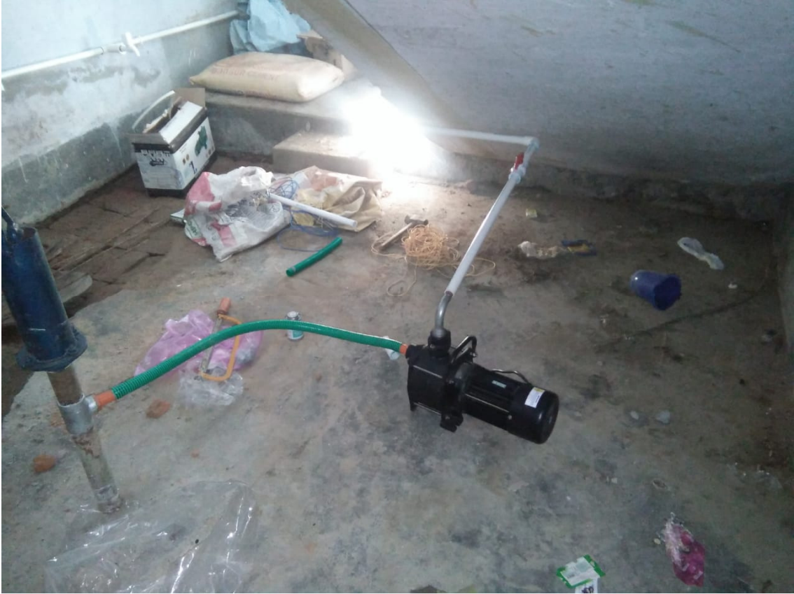
Fitting motor and pipe with tube well
